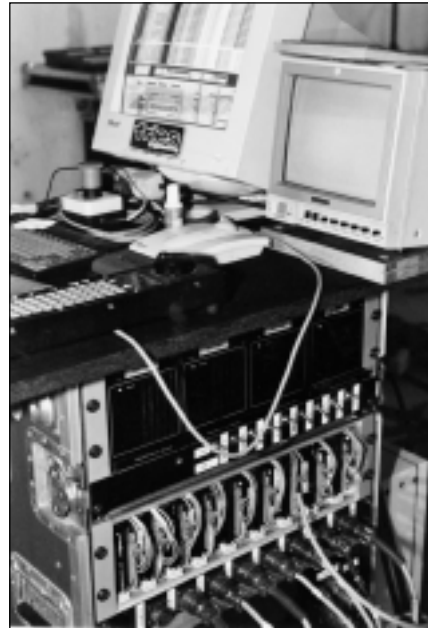
Control console with computer and step motor drivers
